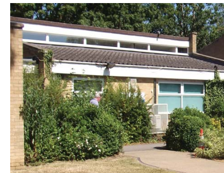
Figure 2.16 Health centre, Exeter Close
