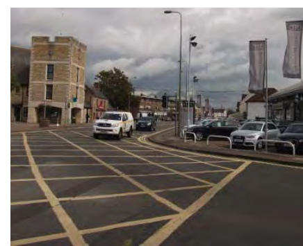
Figure 4.19 Box junction markings dominate the Oxford Road junction
